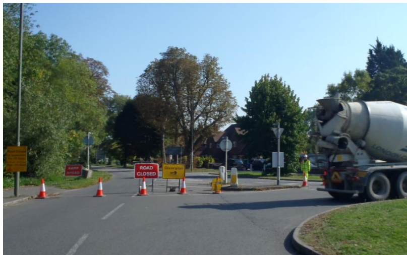
Planned tree works and tree failures will cause traffic disruption
